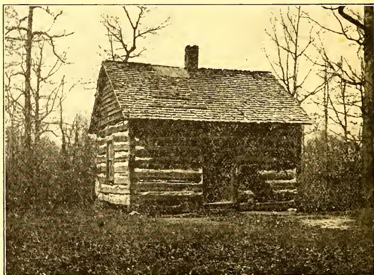
WILLIAMSBURG, No. 3, ROCKINGHAM COUNTY (OLD).
